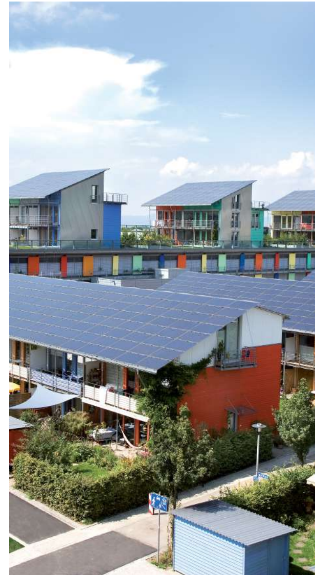
Solar Settlement. © Rolf Disch Solar Architecture, Freiburg, Germany
