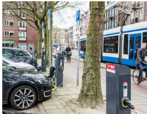
Flexpower Amsterdam project | SEEV4-City: Smart, clean Energy and Electric Vehicles in Amsterdam
