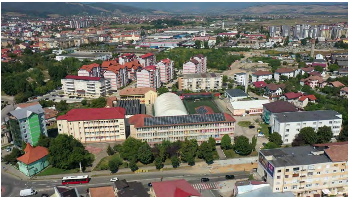
Figure 1. Alba Iulia – PCED core area from above, with the Dorin Pavel Technical School in the foreground, with its 138kW PV installation. Photo by ALEA.
